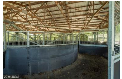
Hot Walker covered by Morton Building
